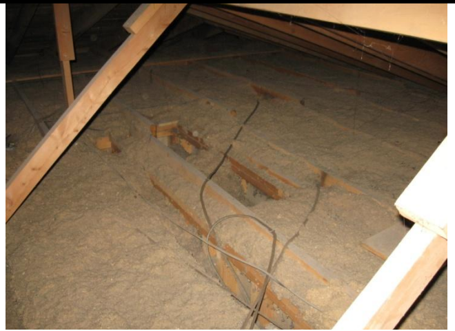
Area between walls needs sealing in attic
