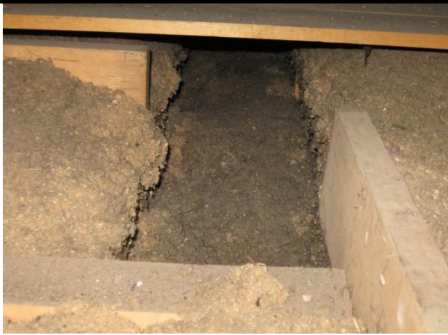
Wall/attic cavity needs filling with insulation
