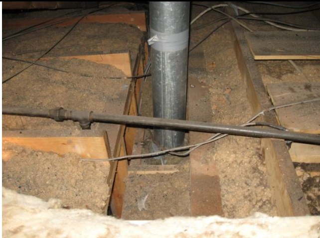
Kitchen drop ceiling soffit needs insulation
